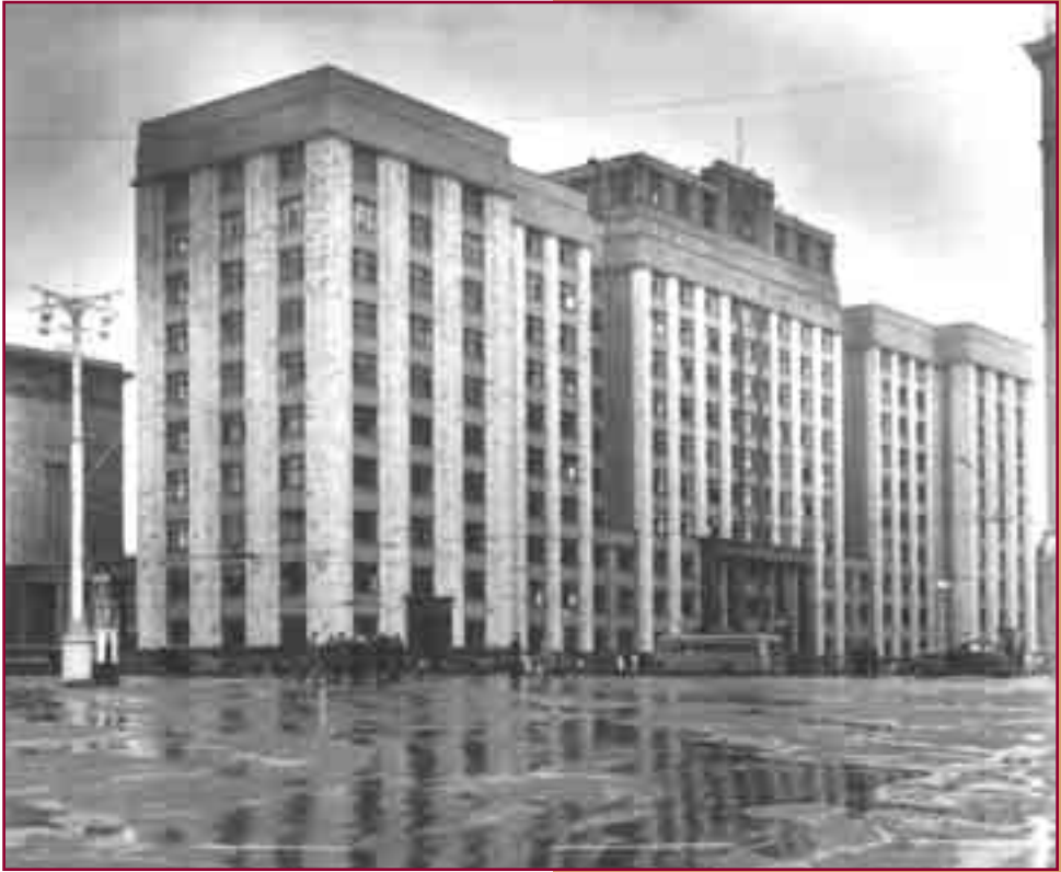
An example of Communism's passion for large buildings: the Building of Council of Ministries in Moscow.
